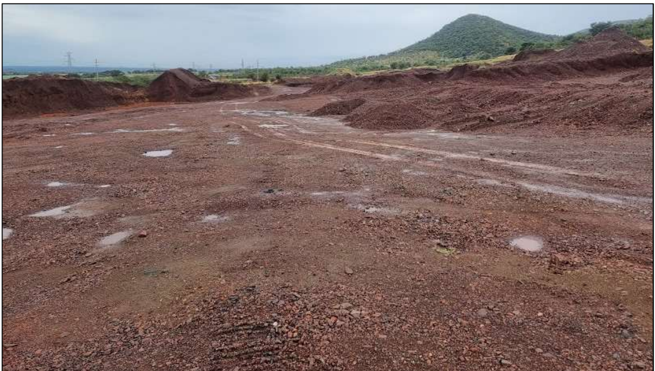
Figure 3: Operational borrowpit active in Site 3. Topsoil historically seems to be consisting of mostly Glenrosa and Mispah soils
